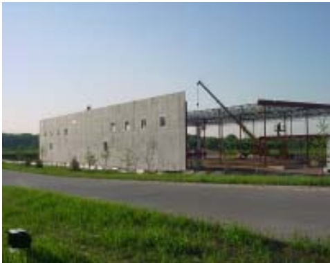
Construction as of June 20, 2005
